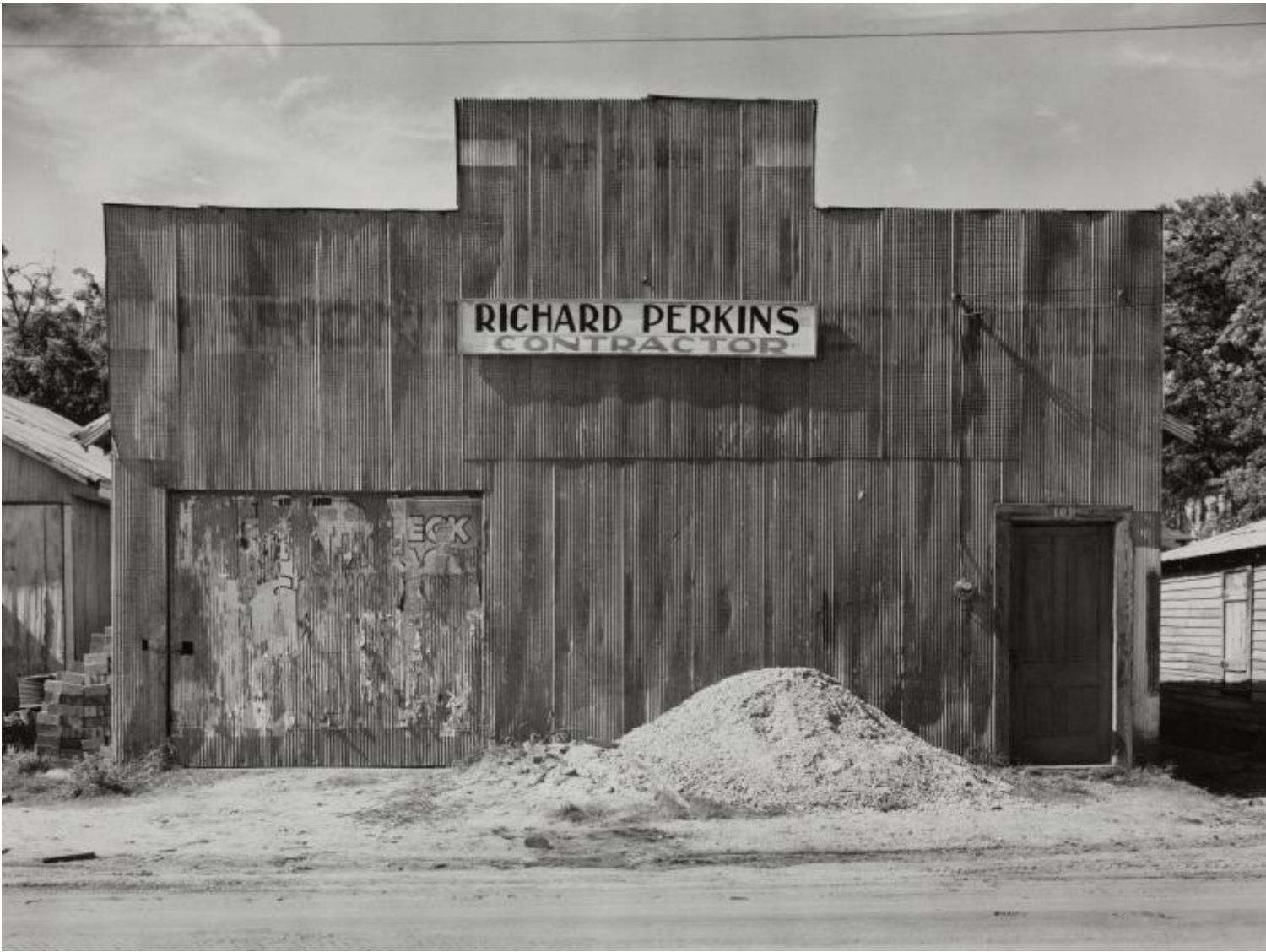
Walker Evans, Tin False Front Building, Moundville, Alabama, 1936
