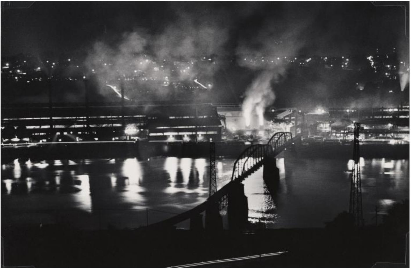
W. Eugene Smith, USA, 1918-1978 Stabilimento National Tube Company, U.S. Steel Corporation, McKeesport, e ponte ferroviario sul fiume Monongahela / National Tube Company works, U.S. Steel Corporation, McKeesport, and Union Railroad Bridge over the Monongahela River, 1955-1957 Stampa ai sali d'argento / gelatin silver print 22.86 x 34.29 cm Carnegie Museum of Art, Pittsburgh Gift of the Carnegie Library of Pittsburgh, Lorant Collection. © W. Eugene Smith / Magnum Photos.
