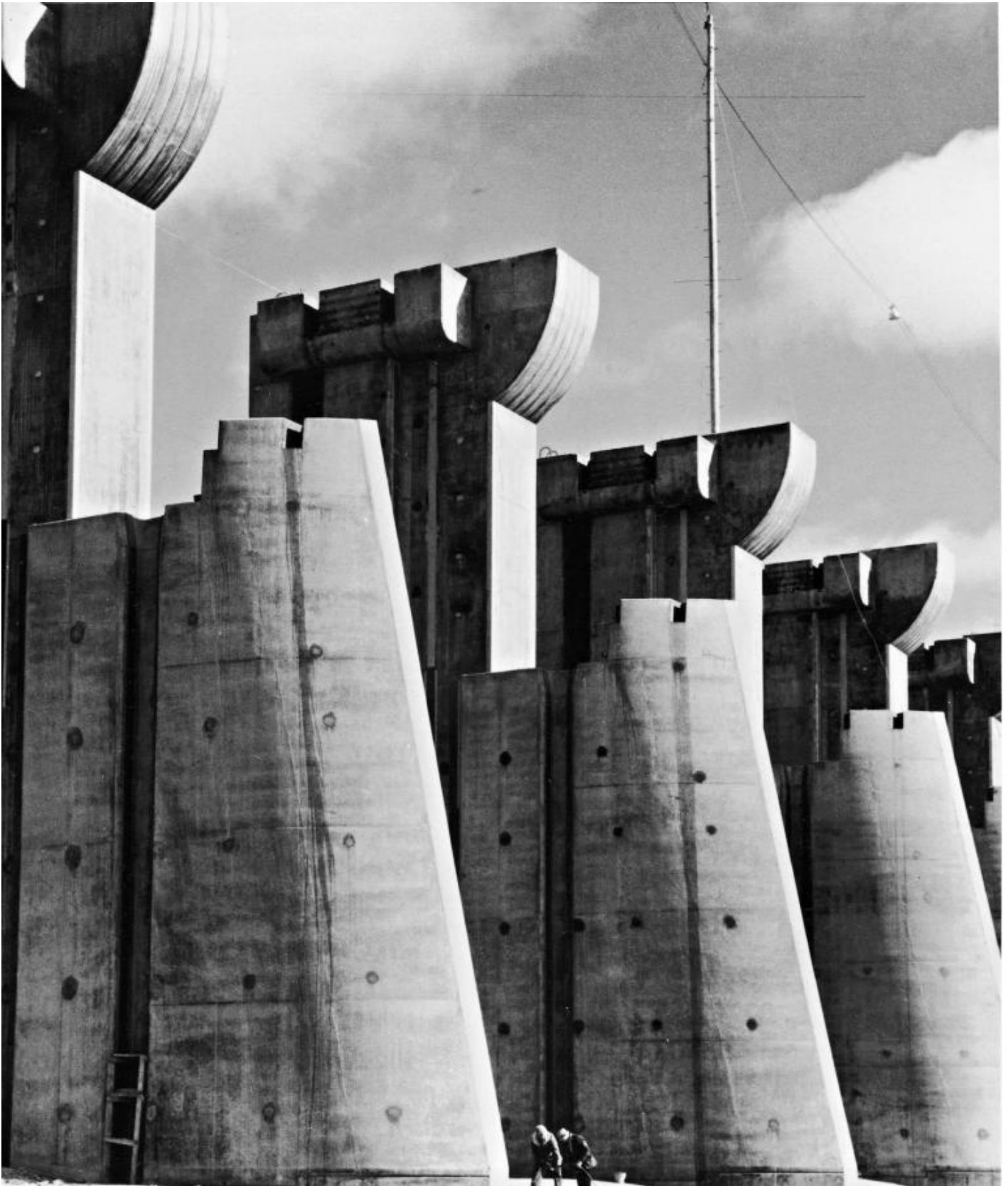
La Diga di Fort Peck, Montana, 1936 . © Images by Margaret Bourke - White. 193 6 The Picture Collection Inc. All rights reserved.
